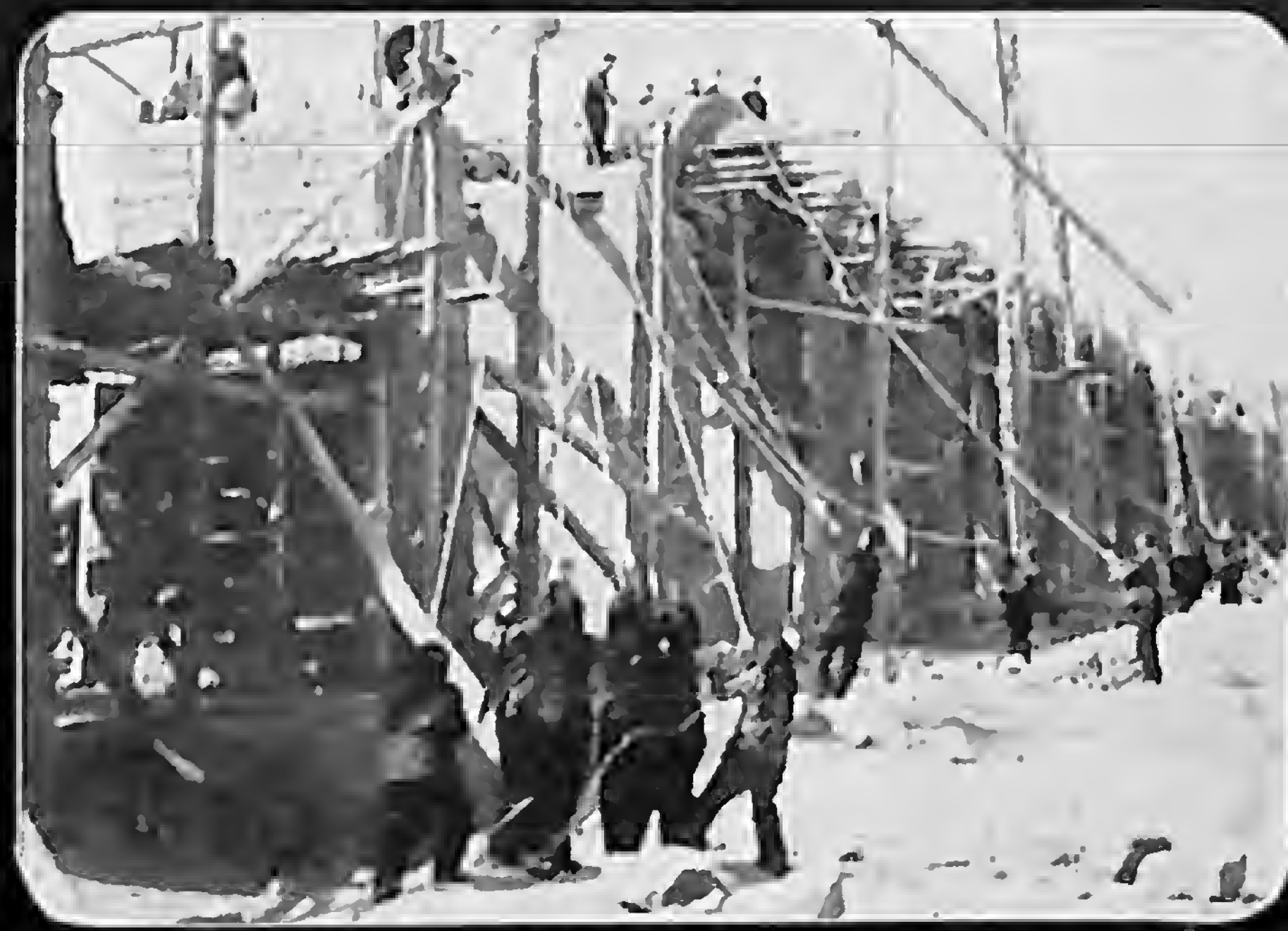
Lifting stones with an improvised derrick.
